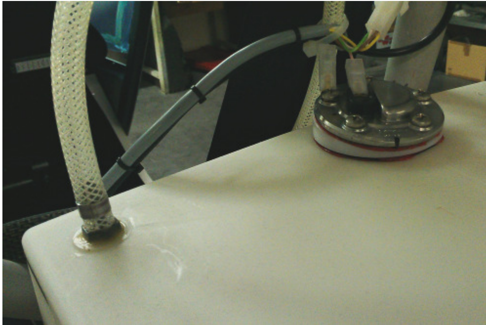
Photo 7: Return line connected
